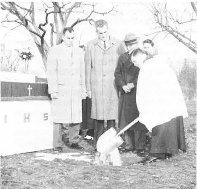
Groundbreaking for new church Thanksgiving Day, 1960
